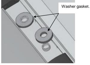
**4:** Place the washer gasket onto protruding plastic tubes in the roof channel.
